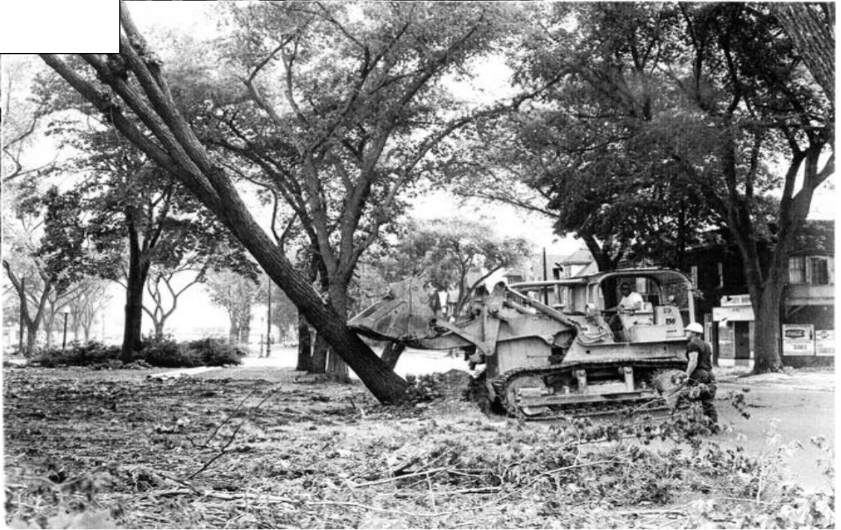
Tree Removal along Humboldt Parkway, 1958 Accessed via the Buffalo History Museum
